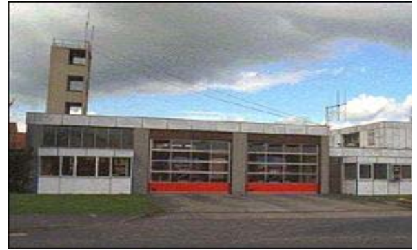
The drill tower has several mobile phone aerials
