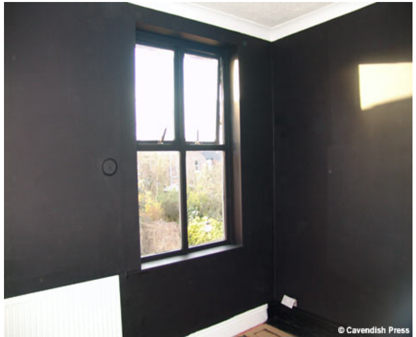
Debbie's home is a radio-wave free zone. A clear protective film has been put on the windows and the walls have been redecorated with a special carbon paint
