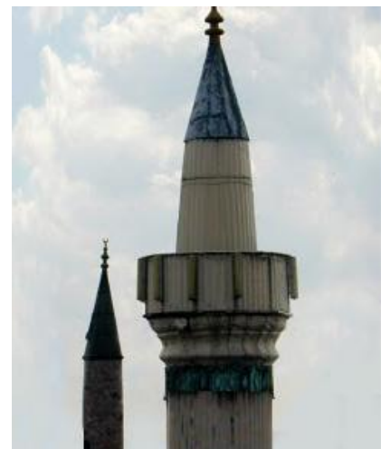
Minaret with relay antennas (add. Next-up)
