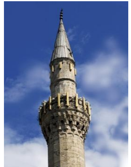
Minaret with relay antennas (add. Next-up)
