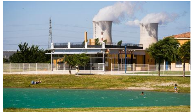
An explosion sparked a fire at the Tricastin nuclear power plant. Some 74% of France's electricity comes from nuclear sources. Photograph: C Brisbois/Fedephoto
