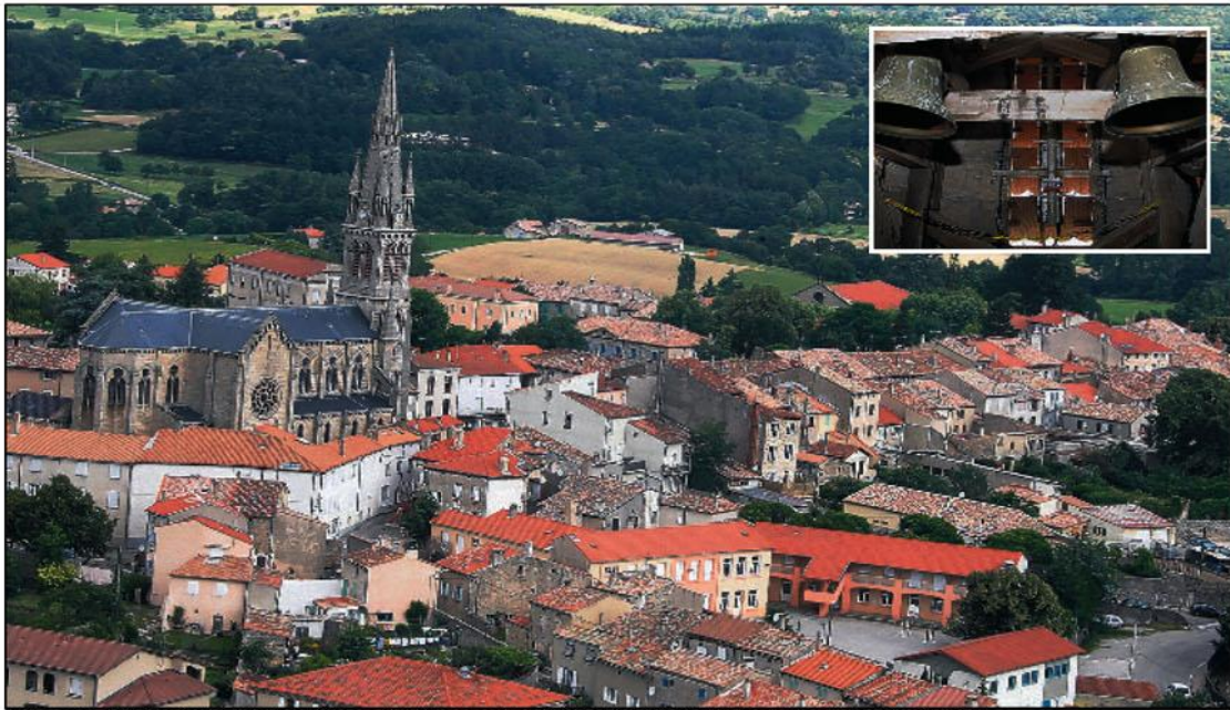
Photo: relay antennas installed in the belfry are cited in a case brought by an inhabitant of Vernoux. Le DL / Fabrice Antérion
