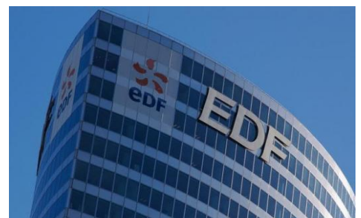
EDF Headquarters in Paris
